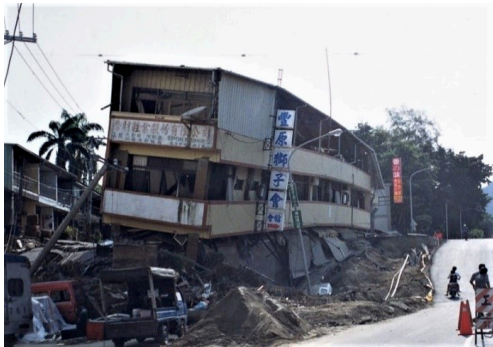
Fig. 2. Damaged buildings above the fault scarp near Chung-Cheng Park, along the northern part of the Chelungpu Fault (October 1999).
