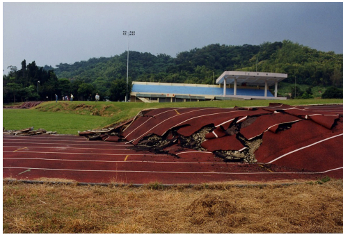
Fig. 1. Looking northward along the surface rupture at Kuangfu Middle School, around the central part of the Chelungpu Fault, there is steep scarp face on the hanging wall over the footwall (October 1999).
